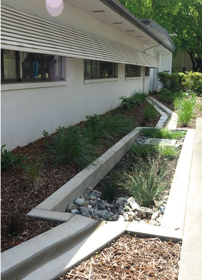
Recent utility projects
