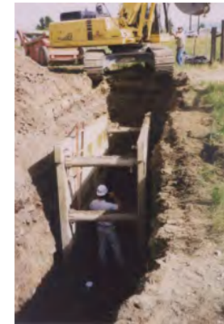
Preparations for Pipe Installation in a Distribution System
