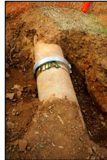
Asset 2: Concrete pipe
