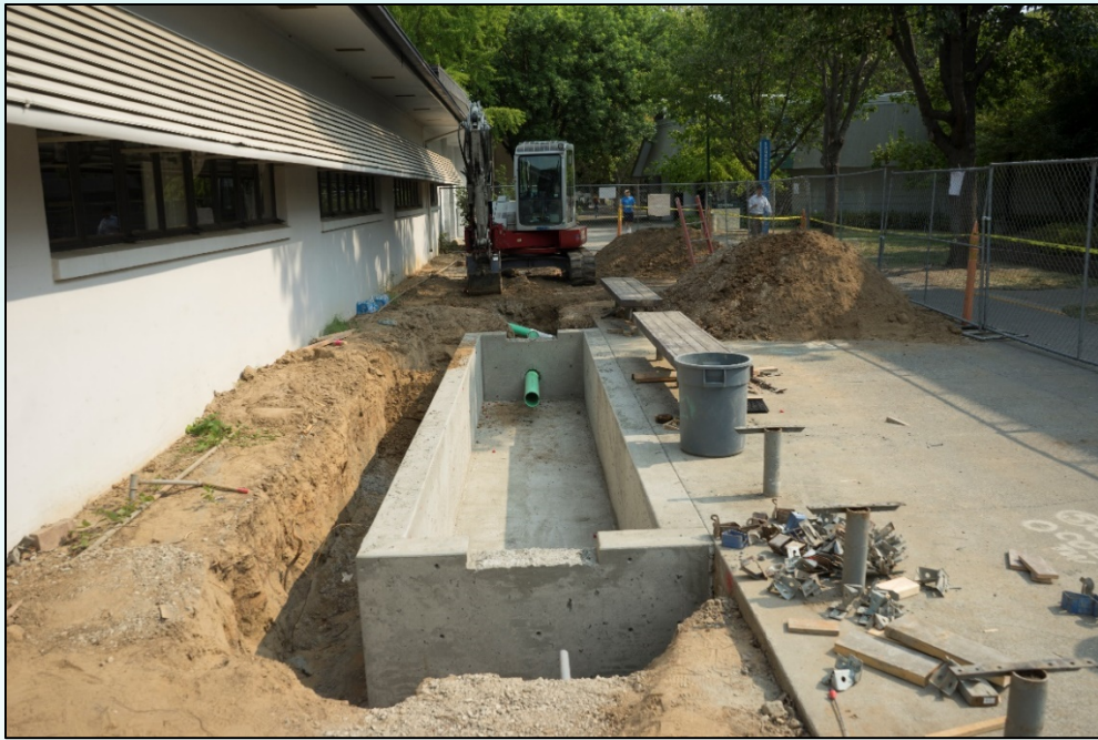
Figure 5: Building a bioretention planter stormwater control measure (Source: OWP)
