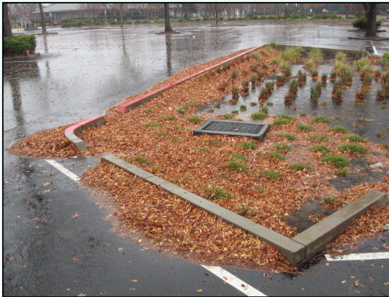
Figure 12: Low impact development device functioning during rainfall (Source: OWP)
