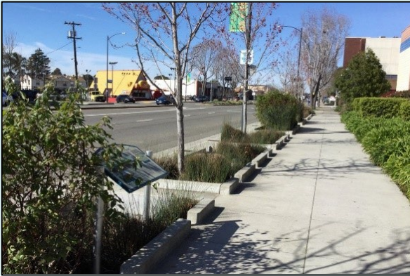
Figure 3: Stormwater capture devices for runoff management: green streets with curb cutouts (left) and infiltration swales (right) (Sources: BASMAA, OWP).
