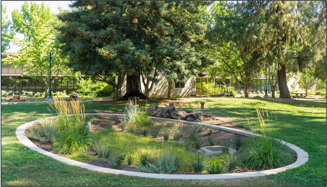
Figure 4: Rain garden stormwater capture device on the campus of Sacramento State University, an example of green infrastructure (Source: OWP)
