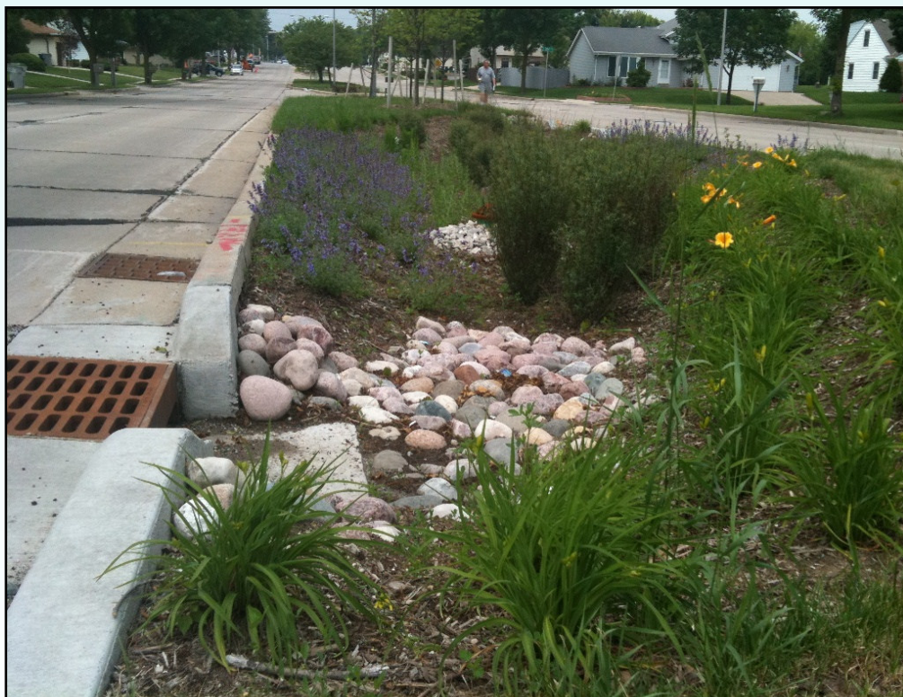
Figure 6: Curb cutout for an infiltration swale (Source: Flickr, Aaron Volkening)
