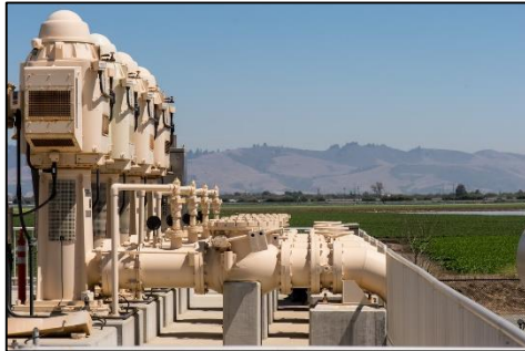
Asset 1: Pumps in station
