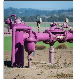
Asset 3: Recycled water pump
