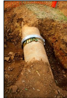
Asset 2: Concrete pipe
